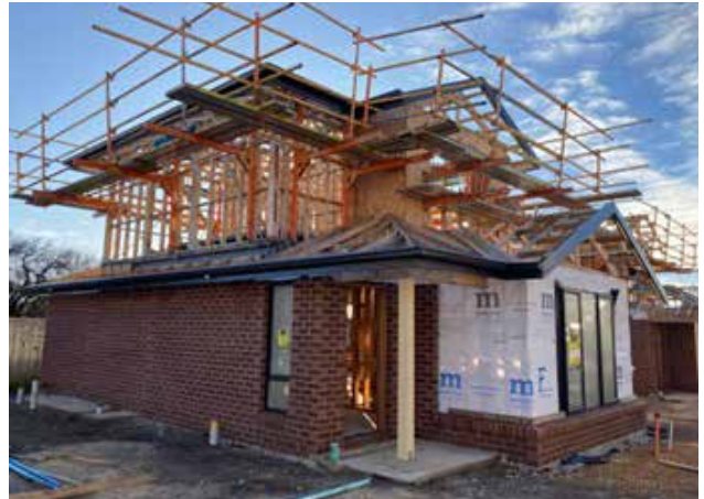
Warrnambool advancing second storey, May 2023
