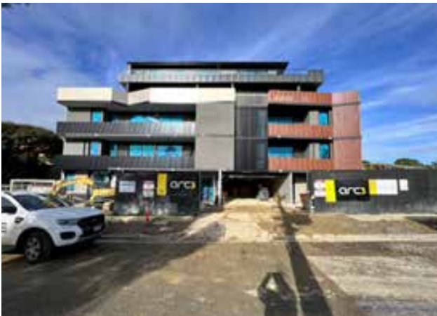
Vermont getting closer to completion in June 2023
