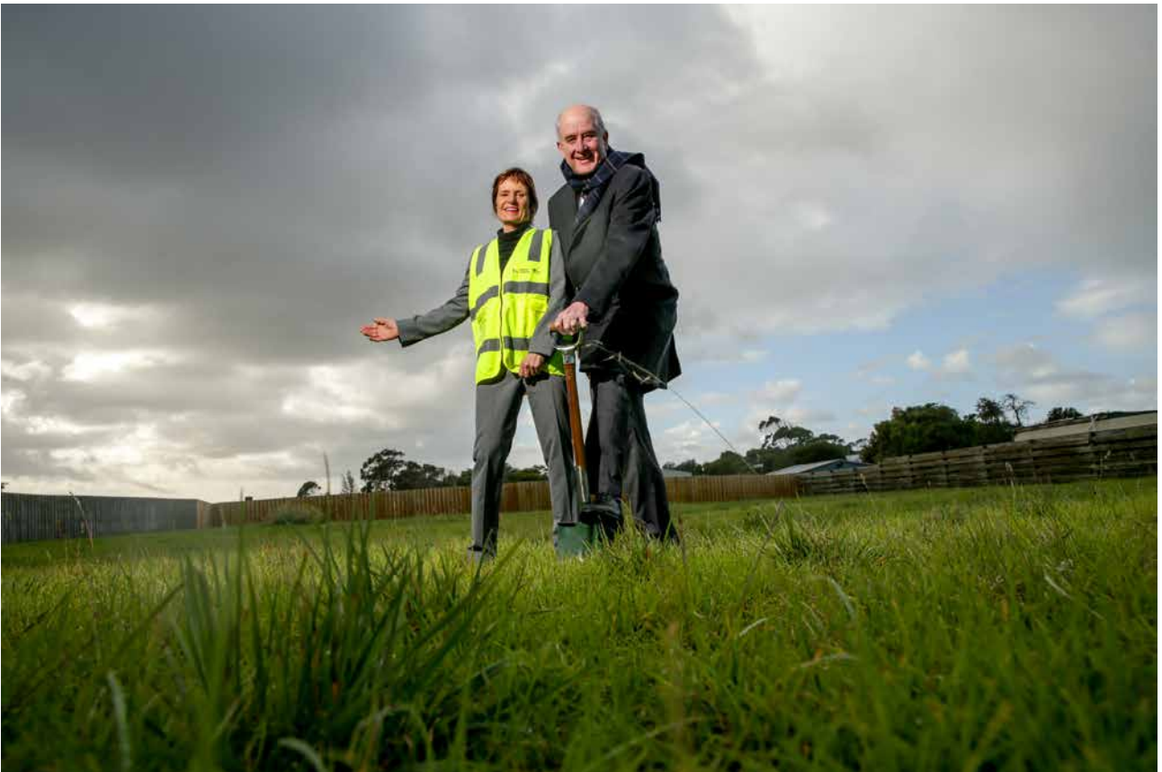
Judy Line, CEO and Richard Wynn, the then Minister for Housing, turning the sod at Warrnambool
